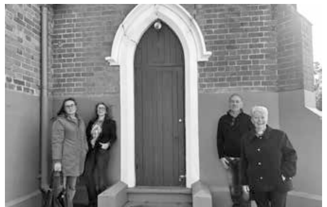
Meckering cracks – Deanna Rokich, Steph Radis, Ward Hellewell and Katrina Holgate stand by cracking caused by Meckering earthquake
