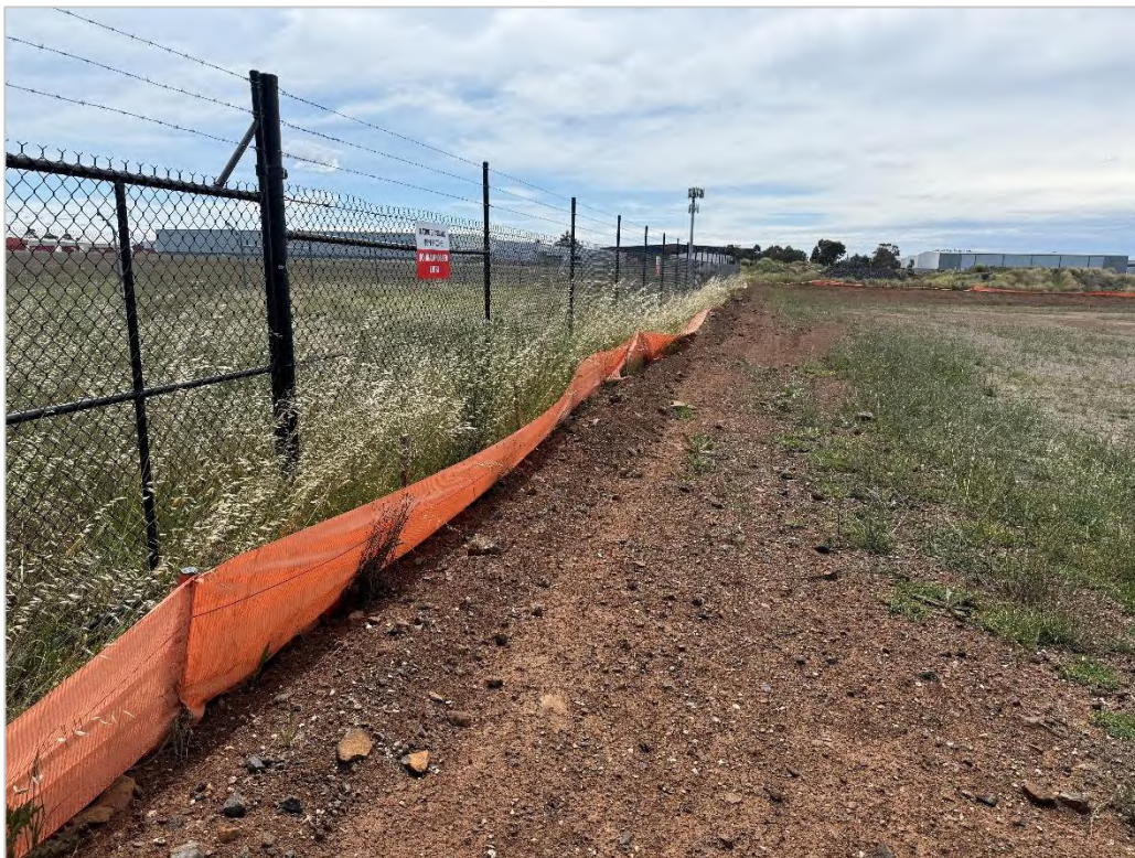
Photo 2: Sediment fencing, occurring adjacent to the buffer zone.
