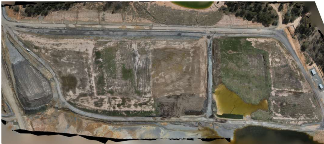
Figure 5-4 Rehabilitation trial area progress (September 2024) aerial image
