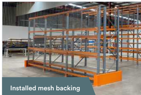
Installed mesh backing
