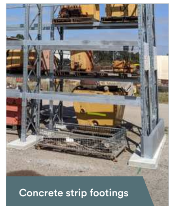
Cross bracing (X-brace)
