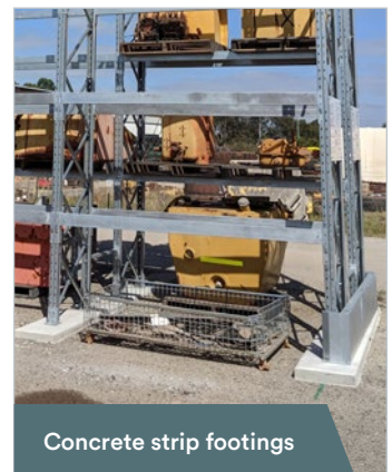
Cross bracing (X-brace)
