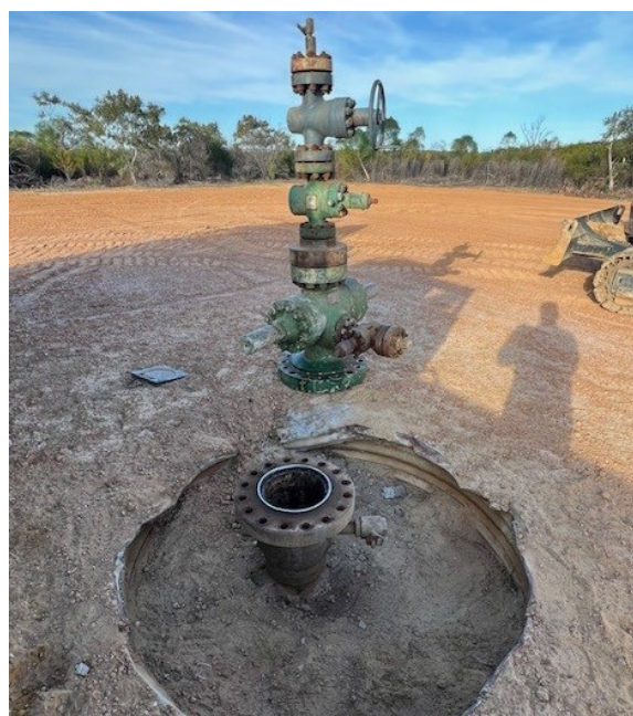
Image: Removal of Woodada 15B wellhead.
