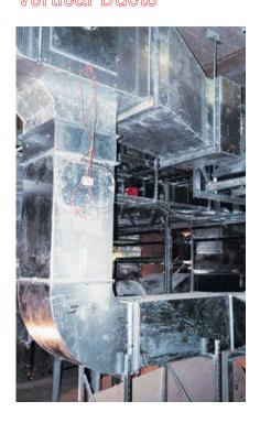
Both DURADUCT SMT and DURADUCT LT systems for all fire performance requirements can be installed in a vertical orientation.
