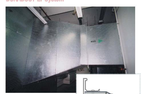
DURADUCT LT is a fast track and economical DURASTEEL® based fire resisting ductwork solution which combines airflow and easy cleaning characteristics of standard galvanised steel ductwork with the armour plated comfort of FIT & FORGET DURASTEEL®. DURADUCT LT is a tried and tested ductwork solution suitable for natural or mechanical ventilation, smoke vents, pressurisation ductwork and kitchen extract ducts.
