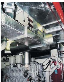
The construction of the DURADUCT SMT insulated system is similar to the DURADUCT SMT system, with the addition of an external covering of mineral wool. This over cladding can perform a number of functions, two of which are:
