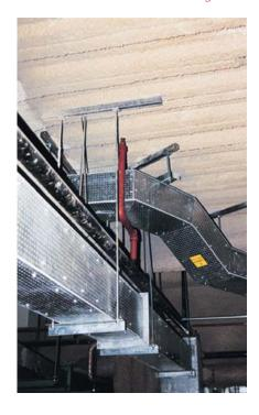
This system is constructed by the fabrication of a steel frame, which is encased in a single layer of DURASTEEL®. The DURASTEEL® thickness will be either 9.5mm for fire resistance periods of up to 240 minutes, or 6mm for fire resistance periods up to 120 minutes in terms of the stability and integrity criterion of BS 467: Part 24: 1987.
