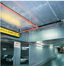
DURASTEEL® horizontal barriers have been fully tested to the requirements of BS 476: Parts 21 and 22: 1987. These barriers can withstand fire exposure from above, below or above AND below, dependent on the design and performance requirements.
