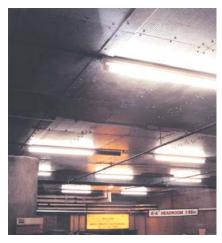
Similarly, double layer membrane ceiling systems can be constructed to cover large expanses with the introduction of additional hanger support systems. Inclusion of these additional supports can often allow a reduction in the dimensions of the support frame members, offering a lighter weight and more cost effective system.
