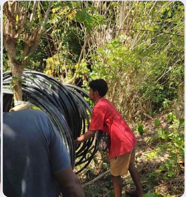
A photo of the Water Project team working with community members to install HDPE pipes.
