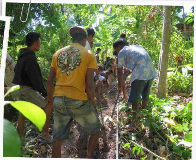
A photo of the socialization activity led by the Water Project team, Pak Cosmos and Pak Simon, along with the initial groundwork involving local residents, including HDPE pipe installation, electricity infrastructure, and main reservoir construction for Palamoko Primary School.
