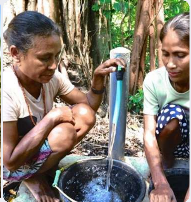
1,2) A photo of community members working hand-in-hand with the Water Project team to dig HDPE pipe trenches, alongside women collecting water from the tap stand (fibertank) provided through our clean water program.
