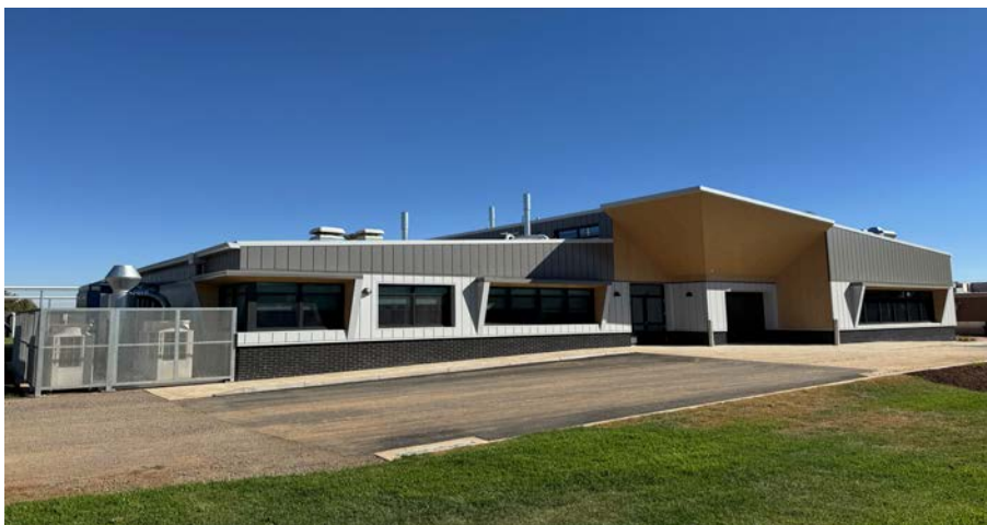
Completed classroom block with the Termimesh System installed
