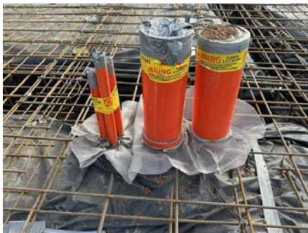
Clustered Termiflange installation comprising multiple pipe penetrations
