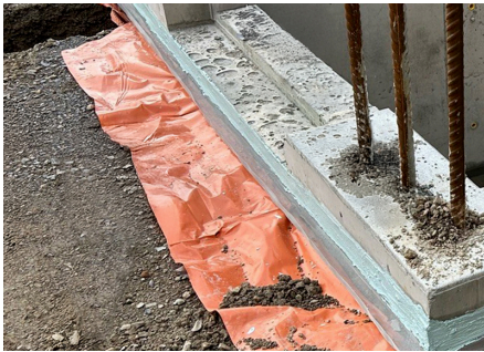
TMA725 stainless steel termite barrier mesh perimeter installation prior to a slab pour
