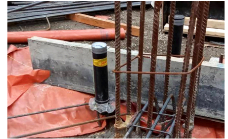
A Termiflange installed around a typical penetration before a slab pour
