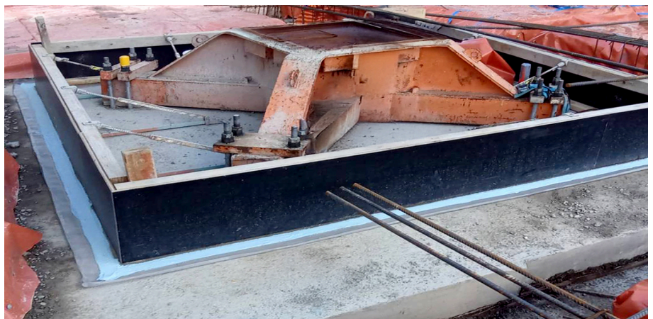
Termimesh installed along the perimeter of formwork prior to the removal of a tower crane base
