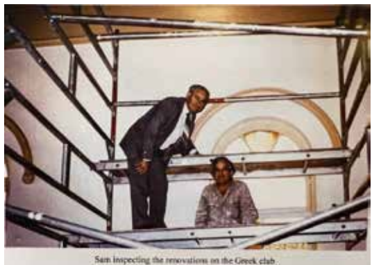
Sam inspecting the renovations on the Greek club.
