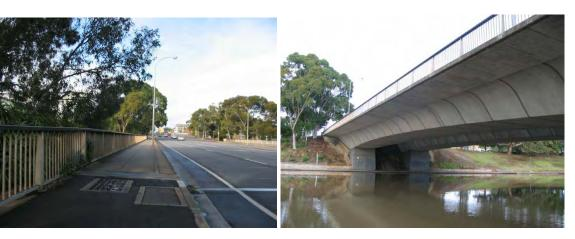
\* Adelaide Bridge: located in the River Torrens/Karrawirra Parri portion of Tarndanya Womma/Park 26, a triple arch reinforced concrete dual carriageway vehicular bridge with Mintaro slate paved pedestrian footpaths, and 2000 erected addition lamp standards on top of the original pylons, opened on 5 March 1931 by state Governor Sir Alex Gore Arkwright Hore-Ruthven and Lord Mayor J Lavington Bonython. Of some engineering and design merit.
