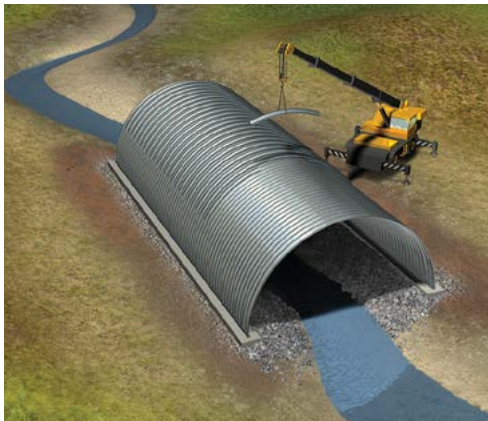
If specified, reinforcement ribs are then added.
