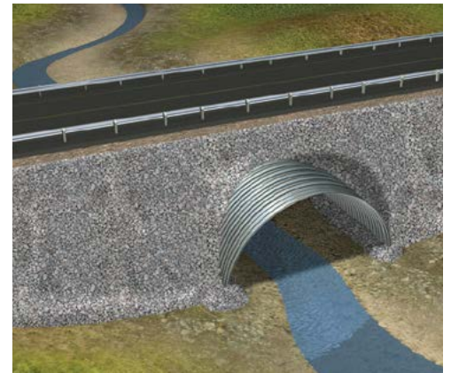
Then the completed road surface is added with safety barriers.
