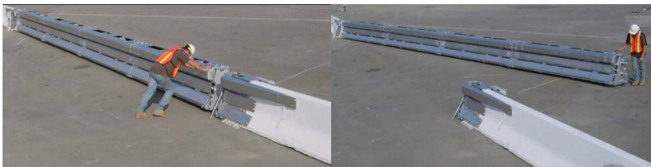
Figure 9 Opening the AGGS System from one end
