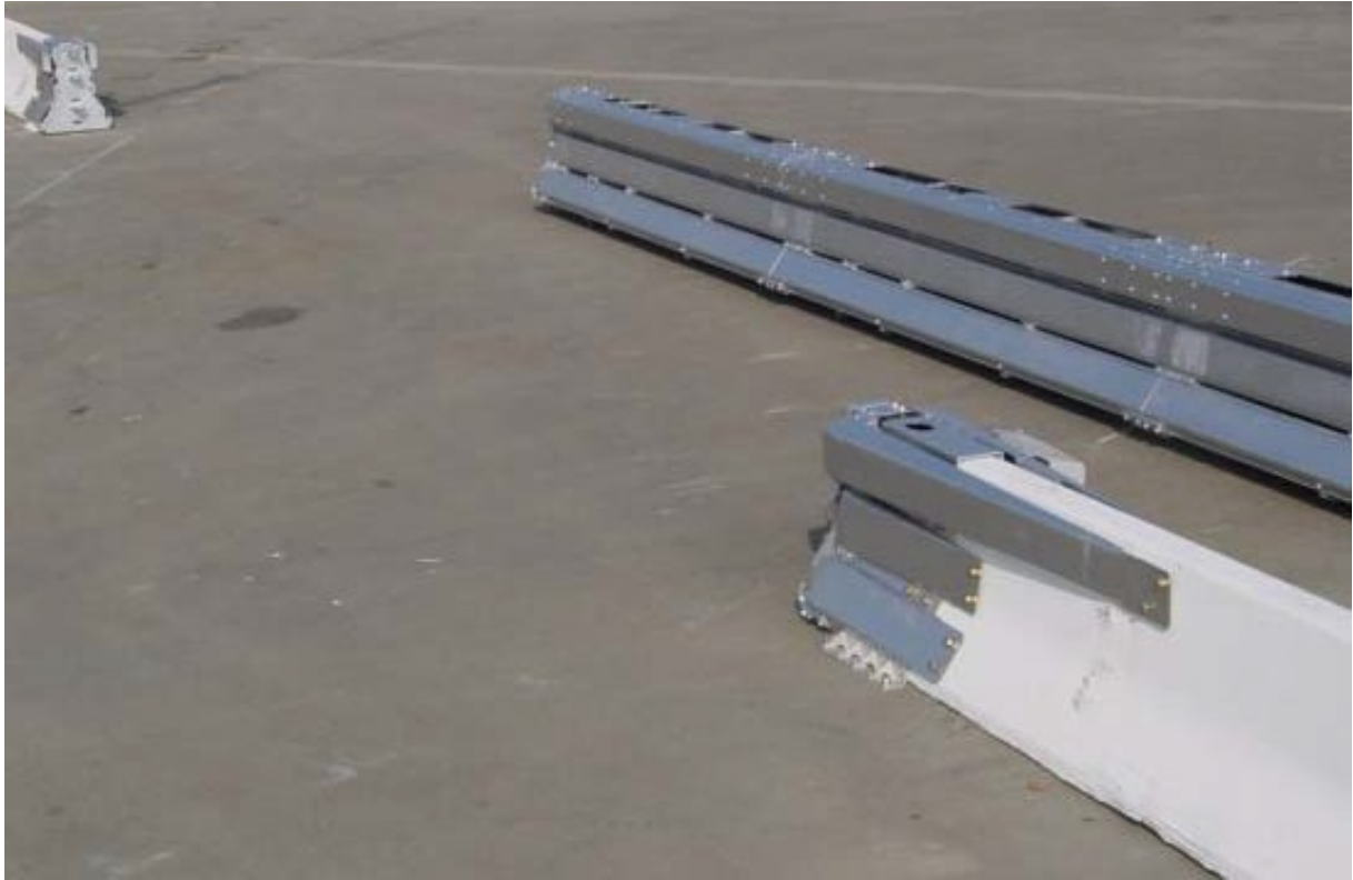
Figure 10 Removing the AGGS System Completely From Opening
