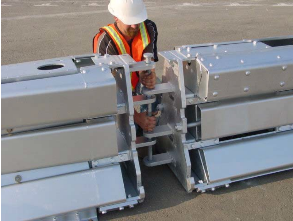
Figure 5 Removing the Main Hinge Pin
