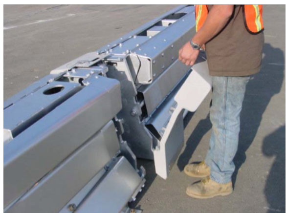
Figure 4 Lift Cover from Hinge Area
