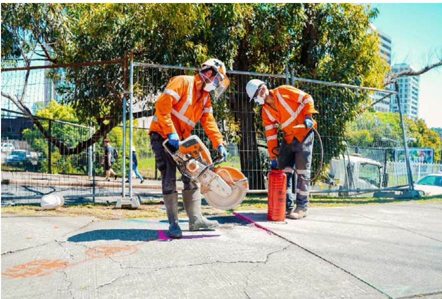
Figure 1-2 Parramatta Connect (Package 4) saw cutting for the Carlingford Bus Shuttle
