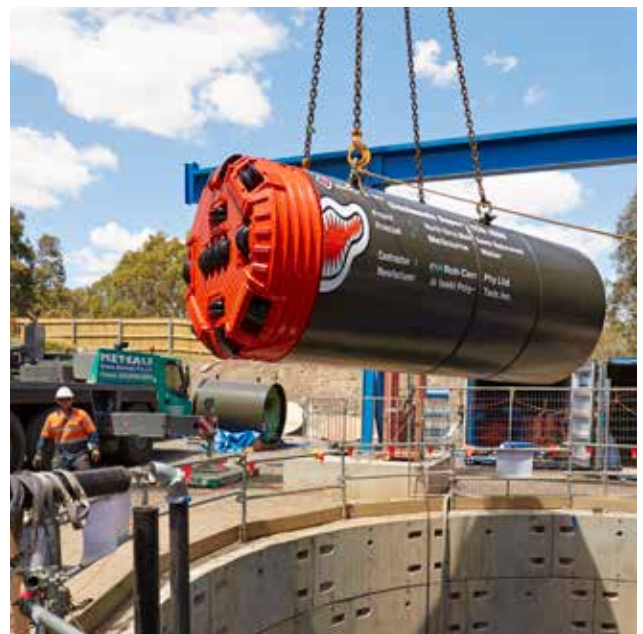
A micro-tunnelling machine lowered into the pit
