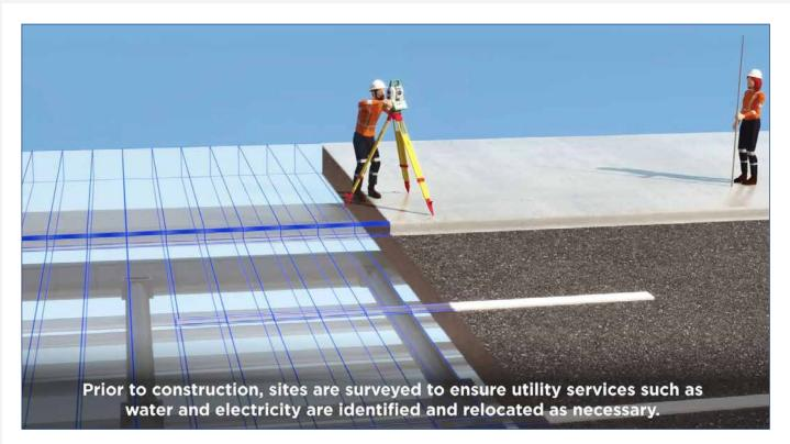
[Words on screen]: Prior to construction, sites are surveyed to ensure utility services such as water and electricity are identified and relocated as necessary.
