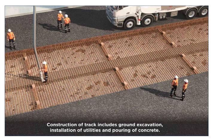
[Words on screen]: Construction of track includes ground excavation, installation of utilities and pouring of concrete.
