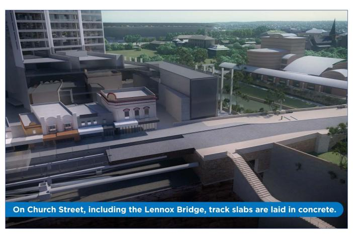
[Words on screen]: On Church Street, including the Lennox Bridge, track slabs are laid in concrete
