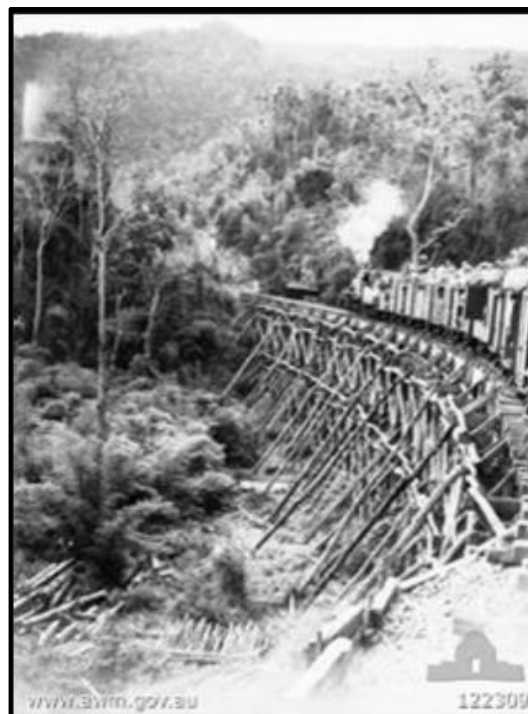
Figure 7: A curved wooden trestle bridge built by POWs, located near Hintok, Thailand.
