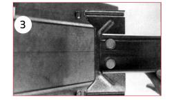
**4.** Fit the other end of the brace into the next purlin. Repeat steps 3 and 4 of the process until the End Brace is bolted to the eave purlin.
