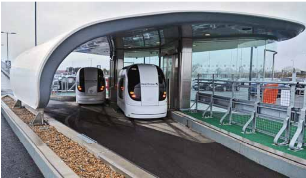
Figure 5 The ULTRA PRT system installed at Heathrow, UK
