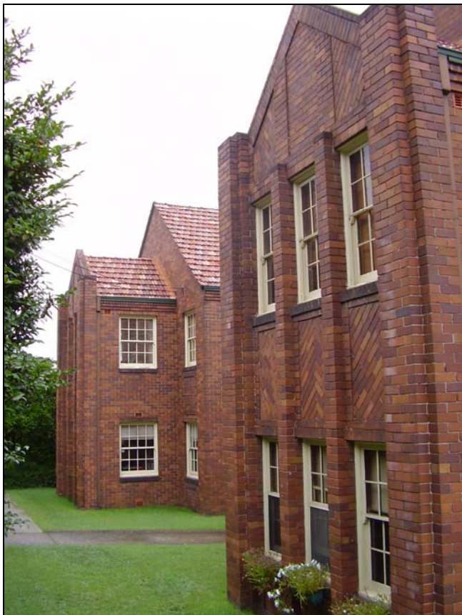
Figure 3.18 No. 4 Epping Road. The two front wings, note the decorative brick detailing.
