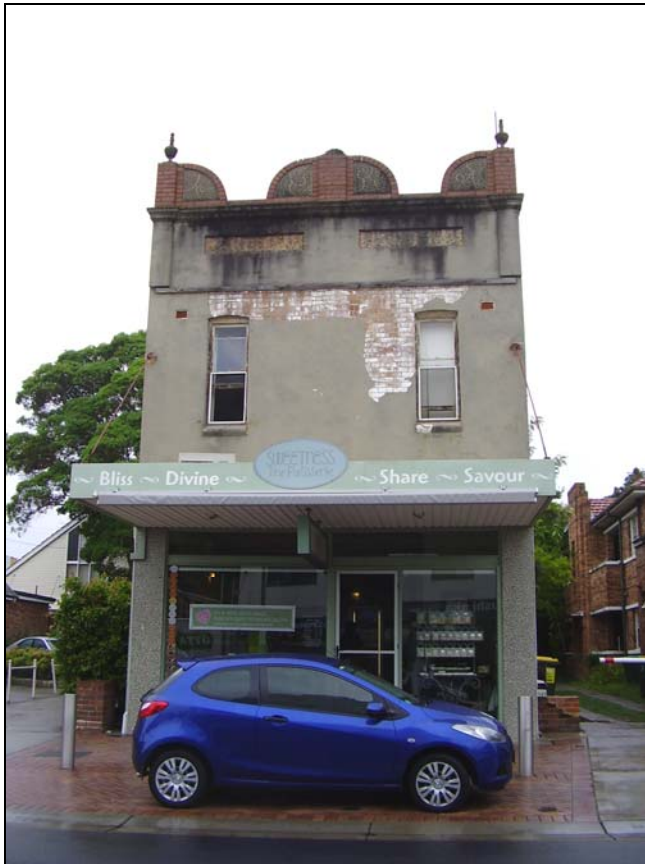
Figure 3.44 No. 38 Oxford Street
