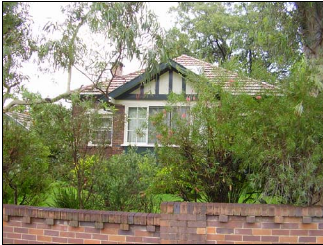
Figure 3.5 No. 9 Cliff Road.
