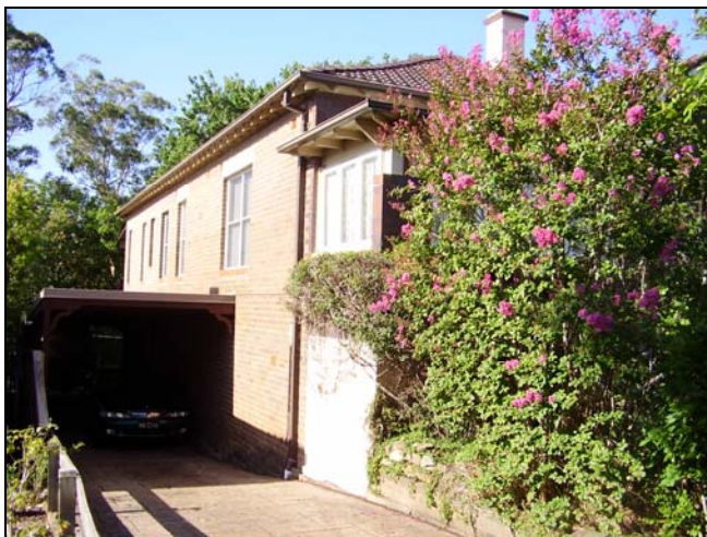
Figure 3.3 Eastern façade and driveway.
