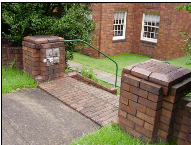
Figure 3.17 No. 4 Epping Road. Detail of the brick piers and stair from the street.
