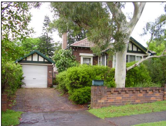
Figure 3.4 No. 9 Cliff Road.
