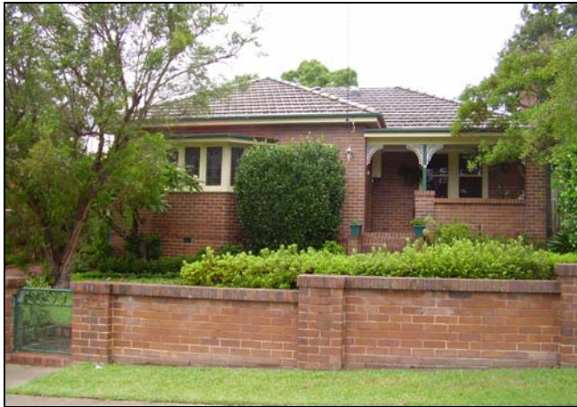
Figure 3.13 No. 19 Cliff Road.
