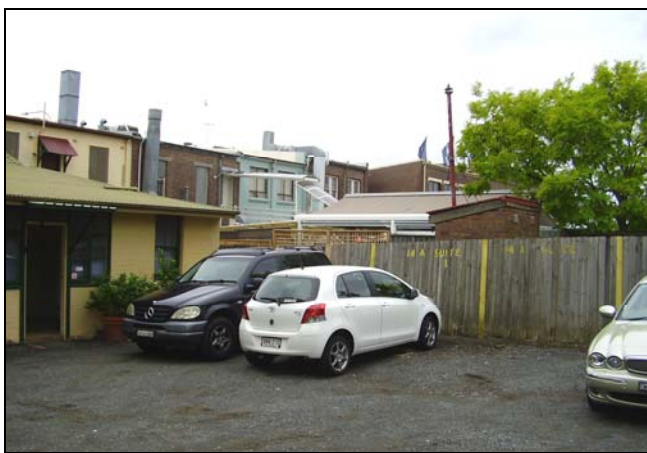
Figure 3.75 Rear of the group, Nos. 2-14.
