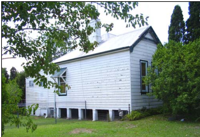
Figure 3.51 No. 91 Oxford Street.
