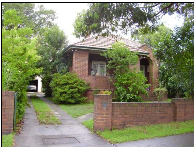
Figure 3.6 No. 11 Cliff Road.
