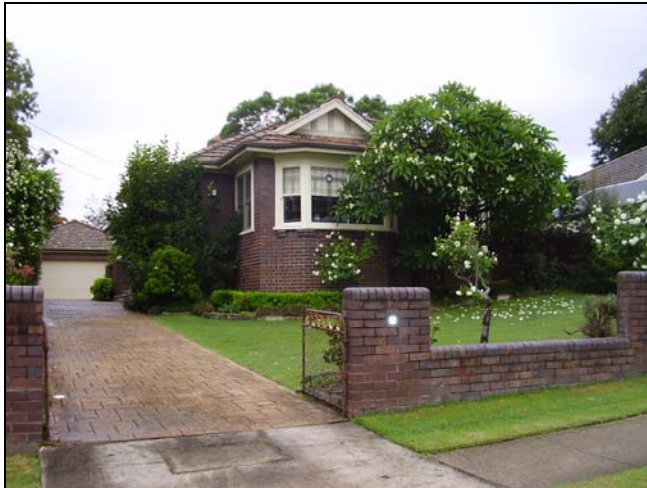
Figure 3.11 No. 17 Cliff Road.
