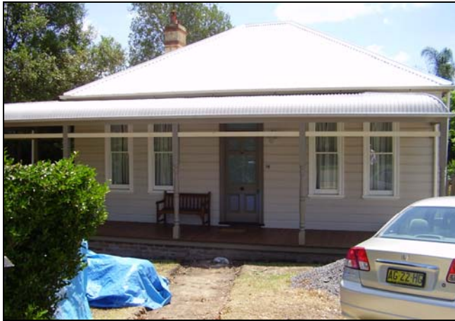
Figure 3.47 No. 85 Oxford Street.
