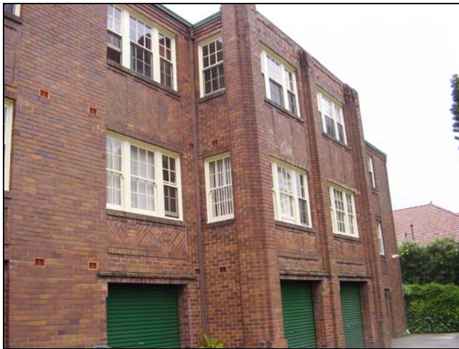
Figure 3.20 No. 4 Epping Road. The rear façade.
