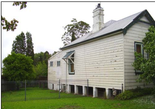
Figure 3.52 No. 91 Oxford Street.
