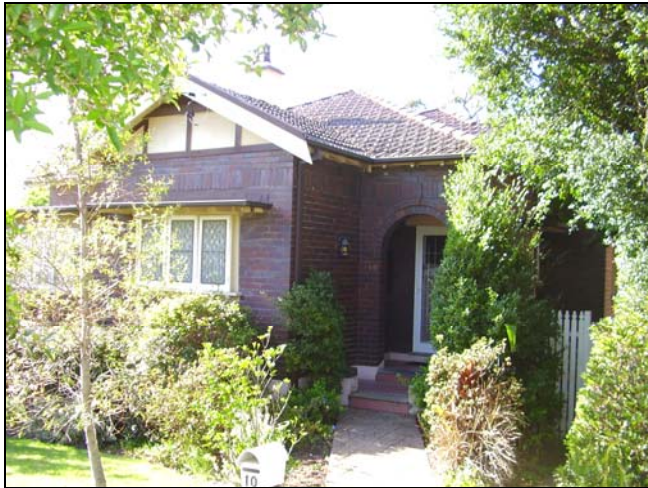
Figure 3.2 Front façade and entry porch.
