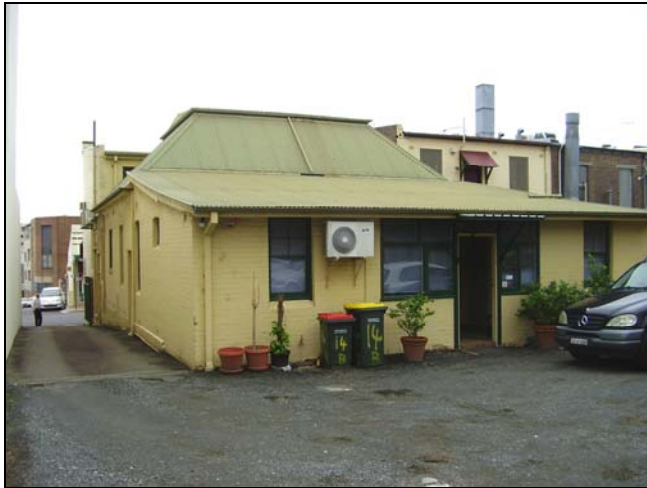
Figure 3.74 Rear of No. 14 Bridge street.
