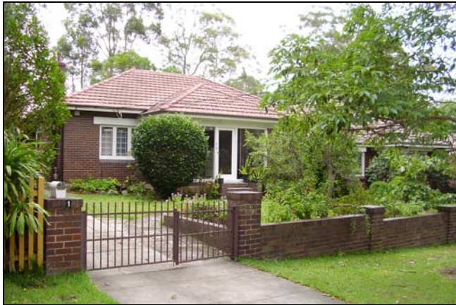
Figure 2.15 No. 1 Rosebank Avenue.
