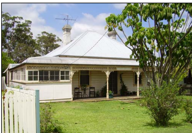
Figure 2.6 Some buildings have undergone some alterations and additions, however, retain their overall scale and character.
