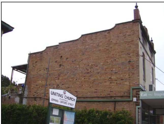
Figure 3.45 No. 38 Oxford Street. Northern façade of the main two storey section of the building.
