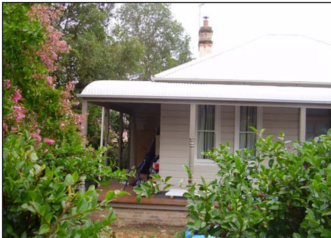
Figure 3.48 No. 85 Oxford Street.
