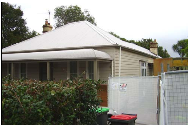
Figure 3.49 No. 85 Oxford Street.
