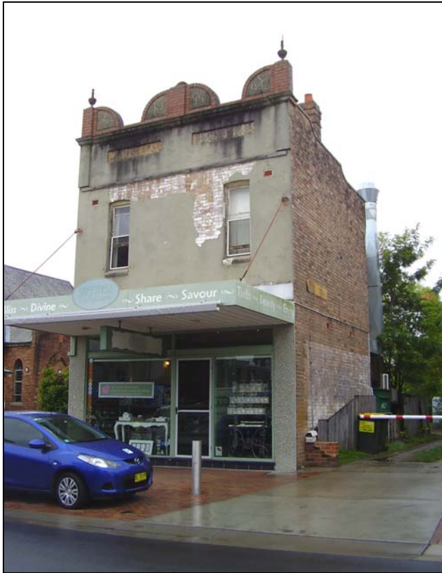
Figure 3.46 No. 38 Oxford Street. Front and part of the southern façade.
