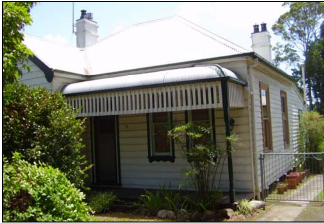
Figure 3.50 No. 91 Oxford Street.
