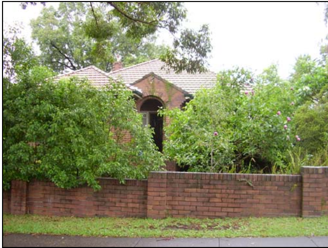
Figure 3.7 No. 11 Cliff Road.
