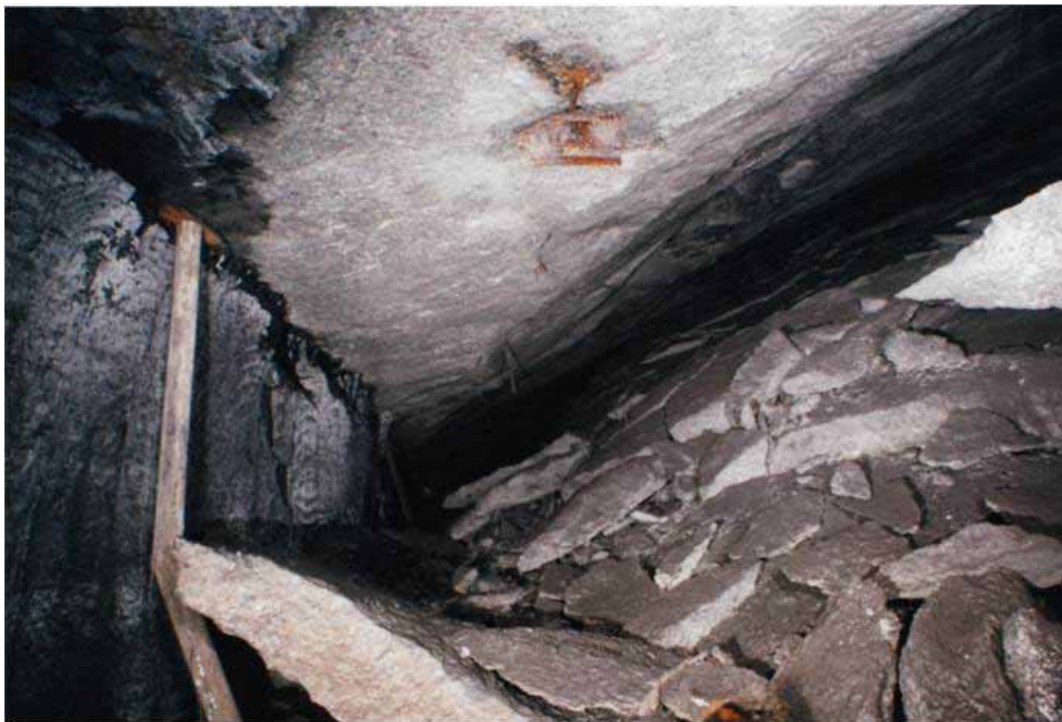
Figure 11: Example of Caving Developing Underground
