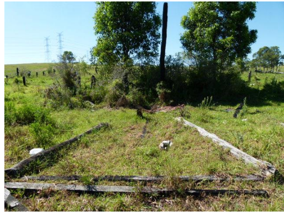
Figure 34: Collapsed shed posts
