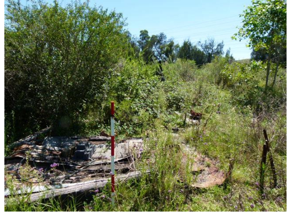
Figure 30: Corrugated iron remains of the long shed
