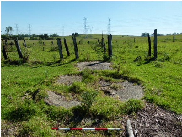
Figure 33: Concrete base for tank
