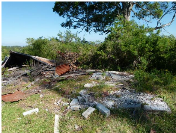
Figure 27: Cottage and bathroom concrete slab
