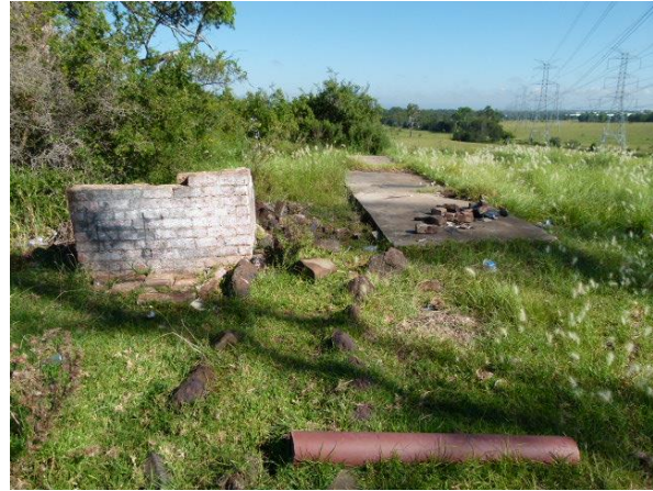
Figure 26: Remains of a chimney and concrete slab structure
