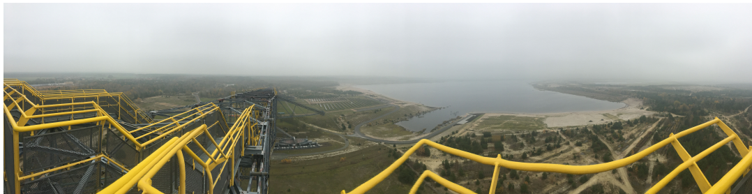
The view from the top of the F60 looking out over Lake Bergheide
