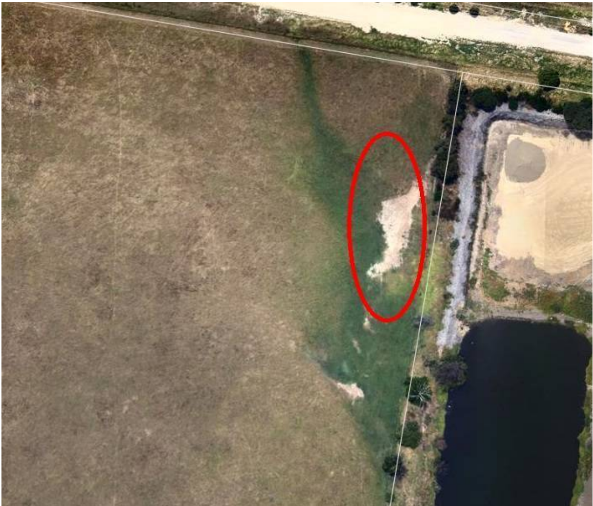
Figure C16: Lot 10 – Suspected washout / erosion of soils from near Lot 102 (February 2011)
