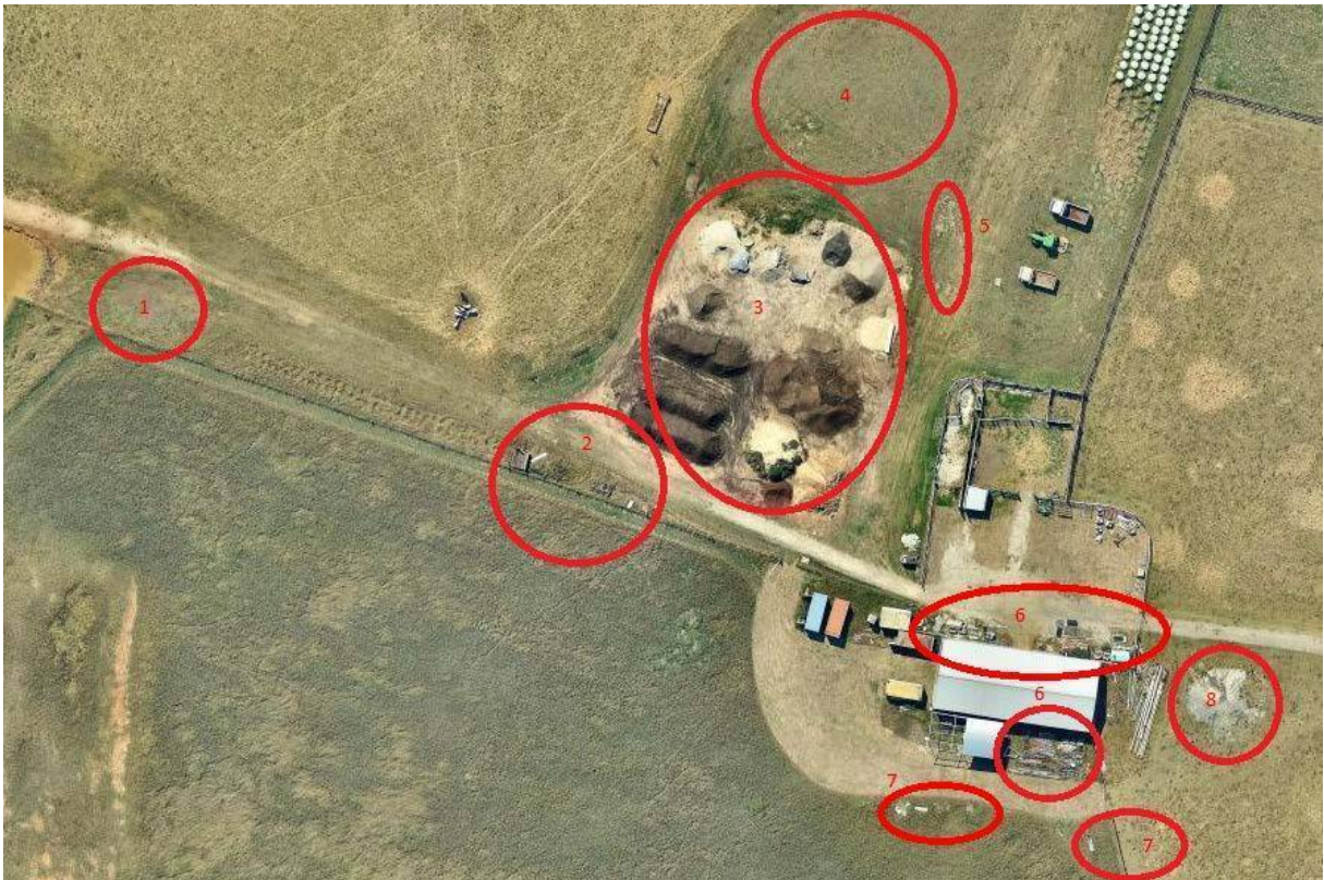
Figure C14: Lot 10 – Unknown features (#2, 4, 5 and 7), stockpiles (#3, 6 and 8) and land scarring (#1) surrounding large shed (October 2011)
