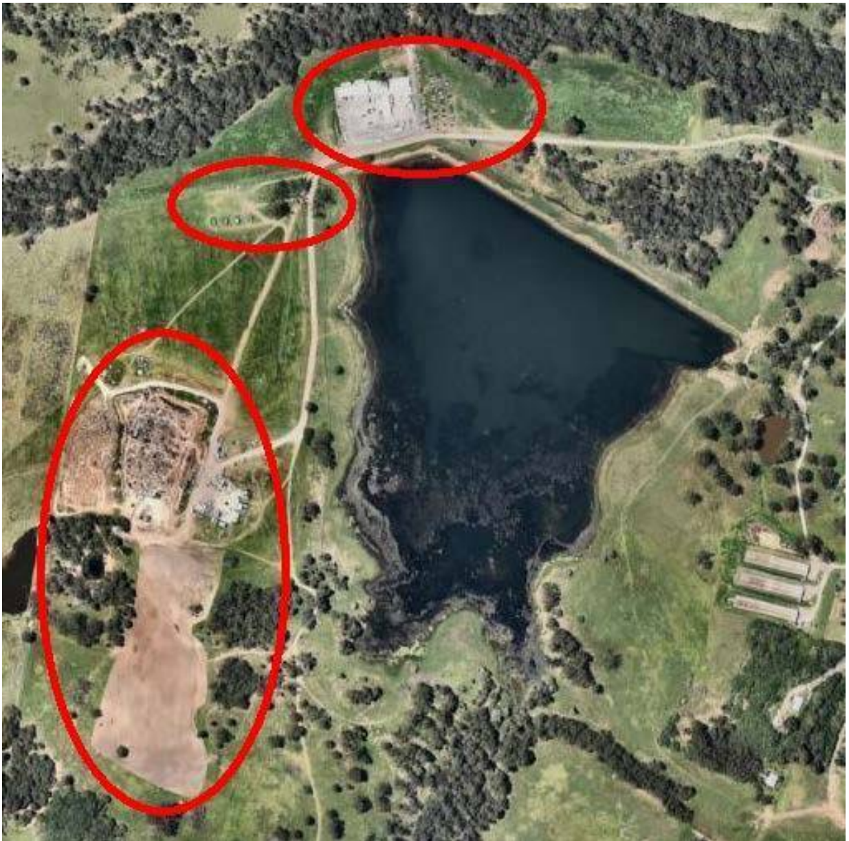
Figure C4: Lot 13 – Land clearance and material storage associated with film set (confirmed by MD to be located at the site during this time) is present at the site (November 2016)
