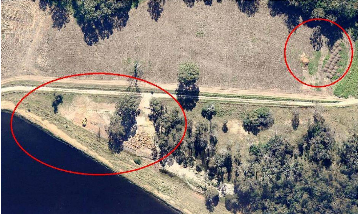
Figure C6: Lot 13 – Land clearing and stockpiling north of westernmost dam (May 2012)
