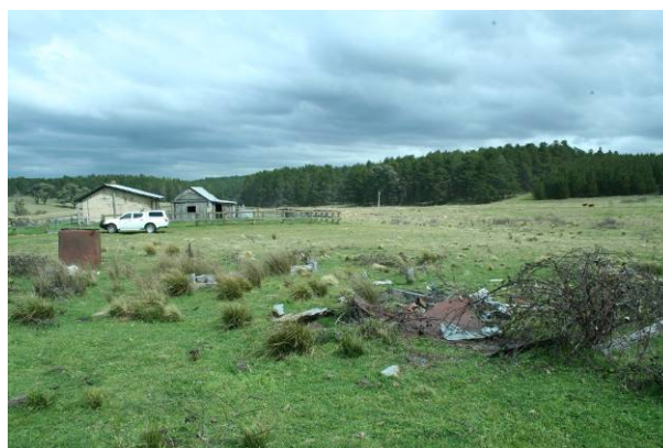
Figure 5 Glenburn Machinery Shed remains in the foreground with pisé and slab cottages in the background (ACT Heritage 2014)
