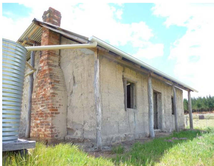
Figure 3 Glenburn Homestead Pisé Cottage southeast facade (ACT Heritage 2013)
