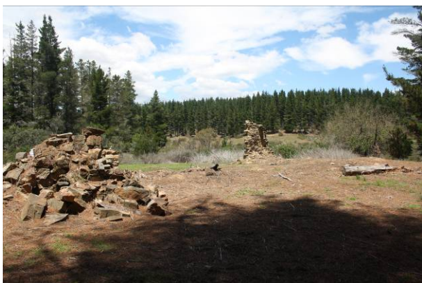
Figure 20 Coppin's Homestead ruin (ACT Heritage 2013)
