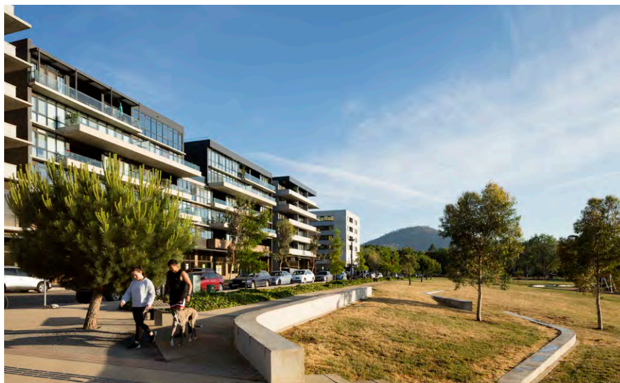
Campbell 5 - heights vary and transition from Constitution Avenue to Campbell Source: Hill Thalix / Photographer: Dianna Snape
