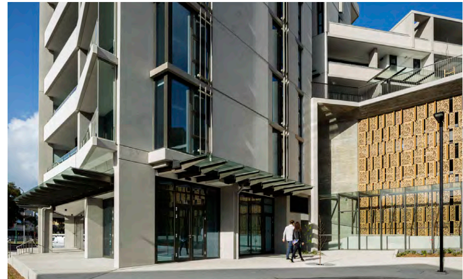
Diversity reflected in building type, orientation and architectural language Source: Hill Thalys / Photographer: Brett Boardman
