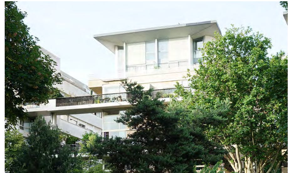
Apartments enjoying the amenity of mature plantings from deep soil in courtyard Source: Hill Thalys
