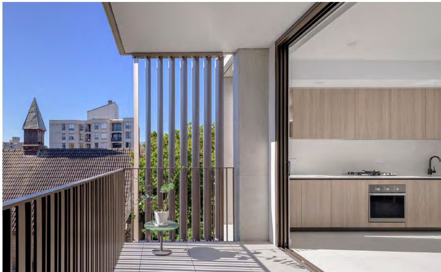
Living areas & balcony receiving optimal sunlight with louvres for summer protection Source: Hill Thalys / Photographer: Ben Guthrie
