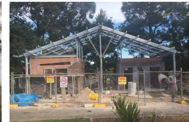
25. changing places toilet (almost complete)
