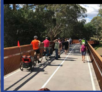
New shared use bridge
