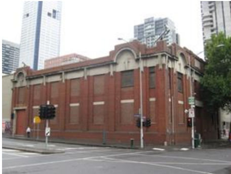
Figure 3. Substation at 651-669 Lonsdale Street constructed 1915.
