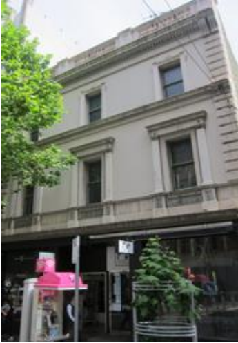
Figure 7. 146-150 Bourke Street constructed 1885. (Source: Context 2018)
