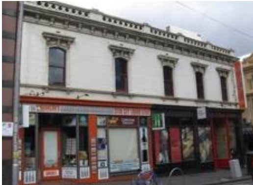
Figure 5. 189-195 Exhibition Street, constructed 1882.
