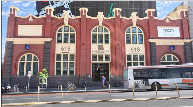
Figure 5. 612-620 Lonsdale Street, built in 1911. (Source: Gogle 2019)
