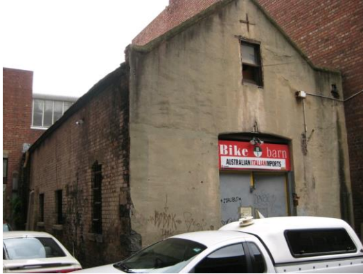
Figure 9. Rear of 361 Little Lonsdale constructed 1854.
