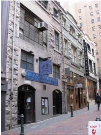
Figure 6. 15-19 McKillop Street constructed 1860.
