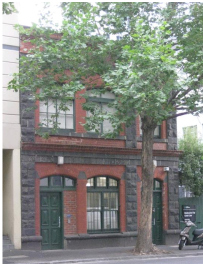
Figure 5. Hoffman's Flour Stores, 104 A'Beckett Street constructed 1851.
