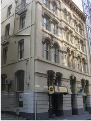
Figure 6. 392-396 Little Collins Street constructed 1882-83. (Source: Butler 2011)
