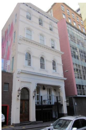
Figure 5. 384-386 Flinders Lane constructed 1885. (Source: Context 2017)
