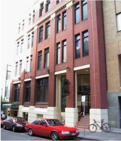
Figure 7. 401-405 Little Bourke Street, built in 1911.
