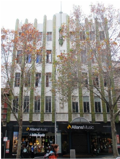
Figure 4. Former Patersons Pty Ltd 152-158 Bourke Street, built in 1934.
