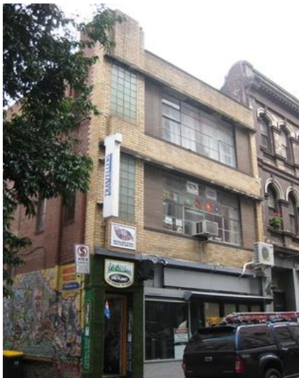
Figure 4. 361-363 Little Bourke Street, built in 1939.
