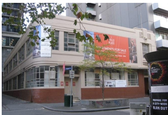
Figure 7. 17-23 Wills Street, built c1930s.
