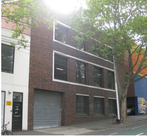
Figure 8. 198-202 Queensberry Street, Carlton, built in 1943.
