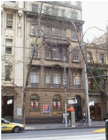
Figure 5. 10-12 Collins Street built in 1916-1925.
