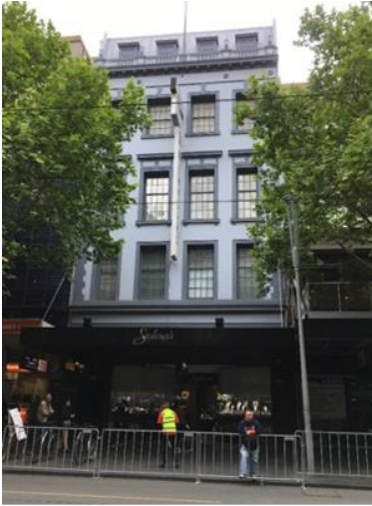
Figure 10. 152-156 Swanston Street originally built in 1888 and remodelled n 1936.
