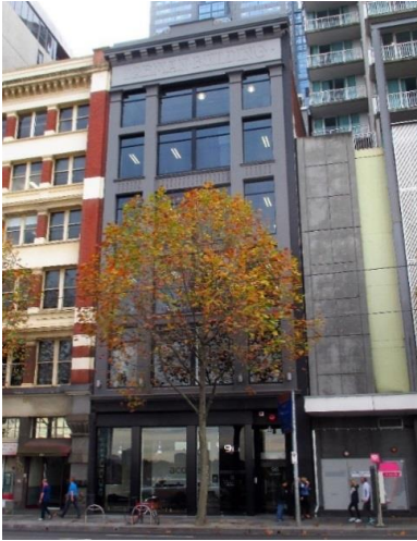
Figure 7. 96-98 Flinders Street, built in 1904. (Source: Context 2017).
