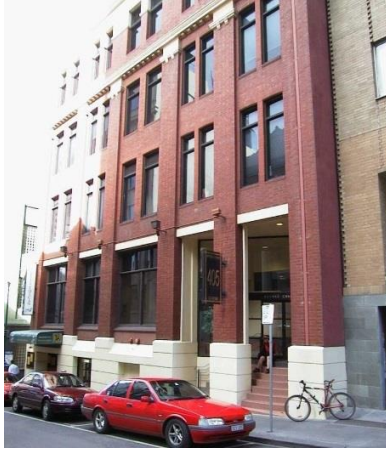
Figure 9. 401-405 Little Bourke Street, built in 1911.
