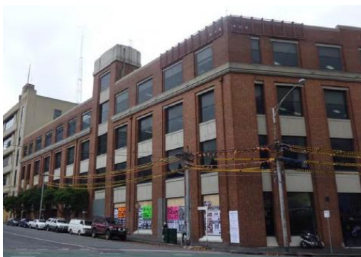
Figure 5. 258-274 Queensberry Street, Carlton, built in 1928.
