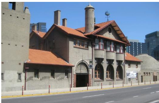
Figure 3. 717 Flinders Street, built in 1937.
