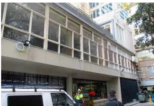
Figure 5. 2-18 Ridgeway Place, built in 1959. (Source: Context 2017)
