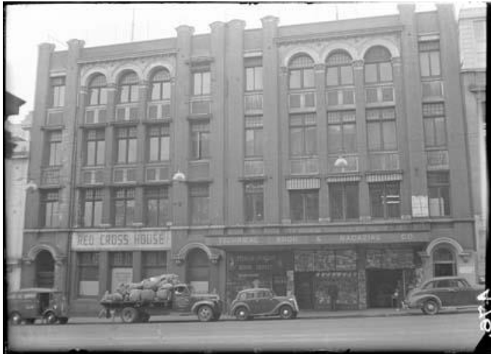
Figure 8. Melbourne Red Cross House, formerly Barnet Glass rubber company (Source: NAA 1917-1968)
