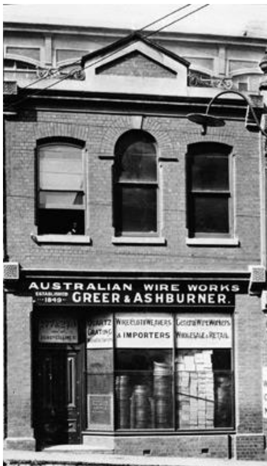
Figure 5. 277-279 Little Lonsdale Street constructed 1903 for Greer and Ashburner. (Source: Clements Langford Pty Ltd, date unknown)
