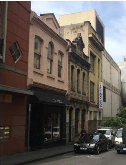
Figure 13. 277-285 Little Lonsdale Street. (Source: Context 2017).
