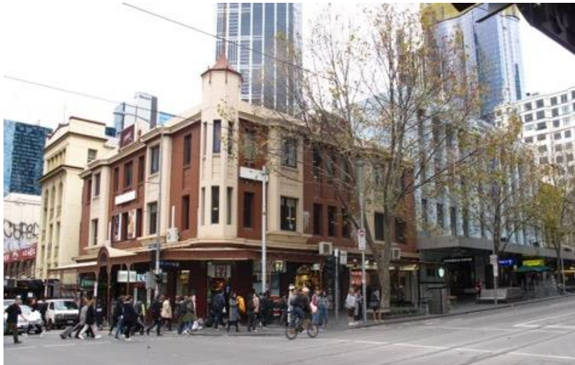
Figure 14. Britannia Hotel Swanston Street. (Source: City of Melbourne, 2018)
