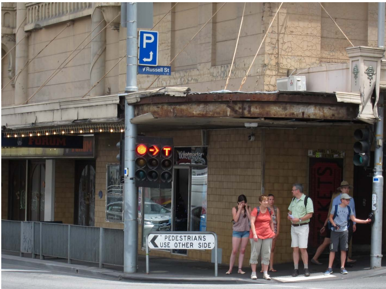
Figure 13: Missing pedestrian crossing point on the corner of Russell and Flinders Streets
