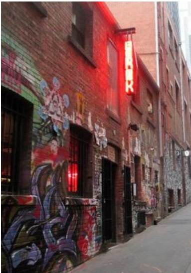
Figure 7. 11-15 Duckboard Place constructed 1885-87.
