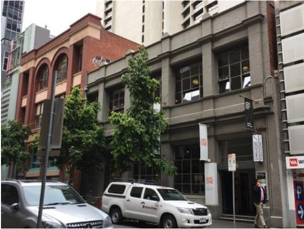
Figure 6. 37-45 Flinders Lane. (Source: Context 2017)
