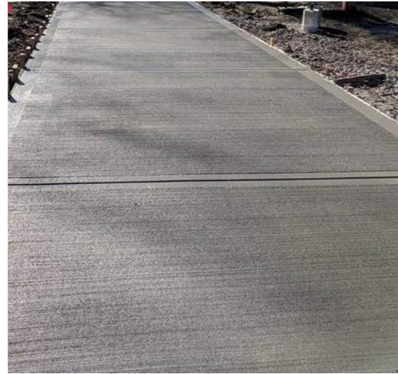
Broom Finished 2.5m Concrete Path
