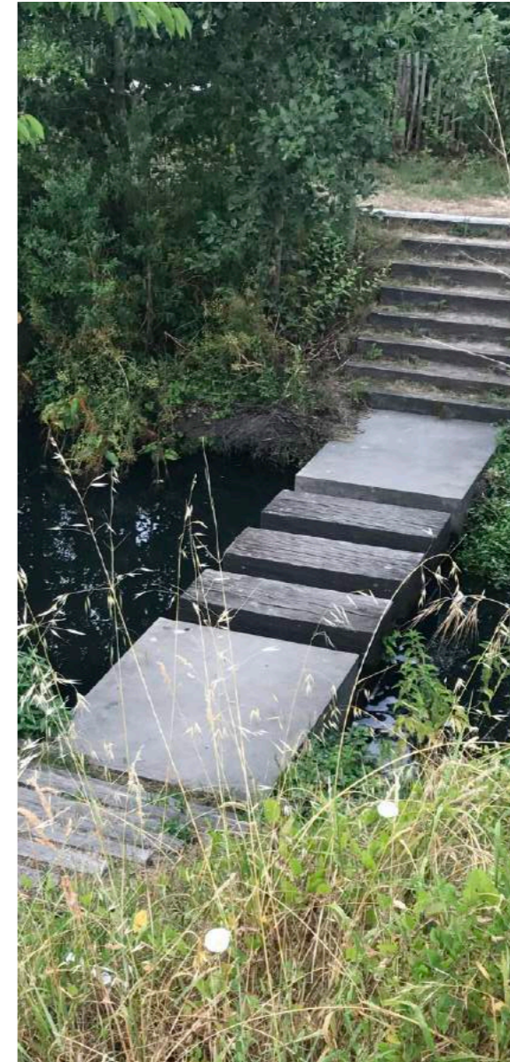
Concrete Stepping Structures
