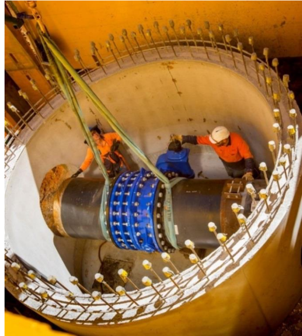
Valve installation at one of the new pits
