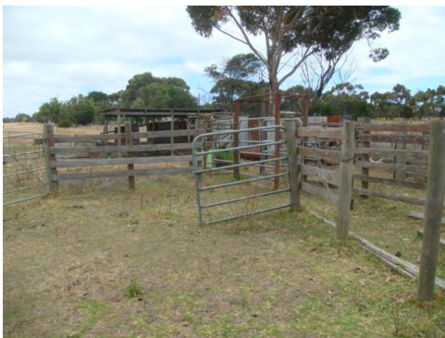
Plate 7.3 : Example of a stockyard structure
