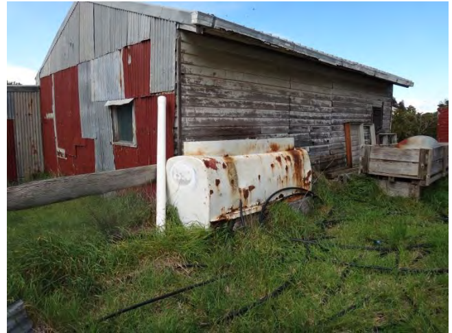
Plate 7.6 : Fuel storage tank at property 2
